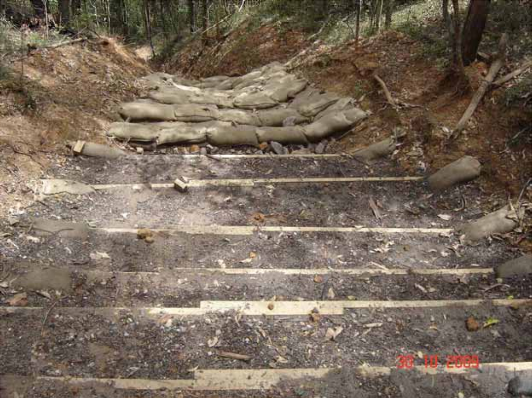
Sandbags filled with soil and fertiliser at the end of the gully
